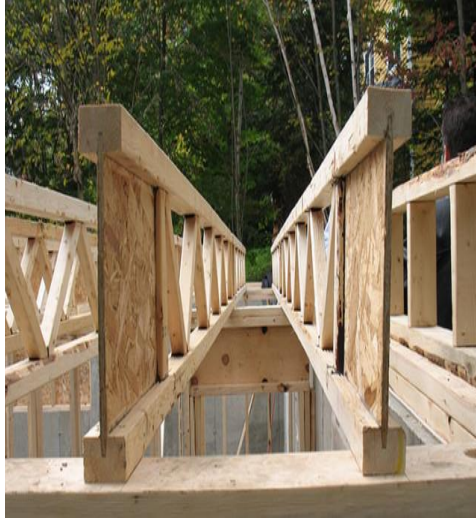
Figure 5.12 Triforce Joists
